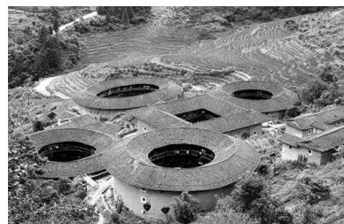
图 1 客家民居建筑群 Fig.1 Hakka residential buildings
